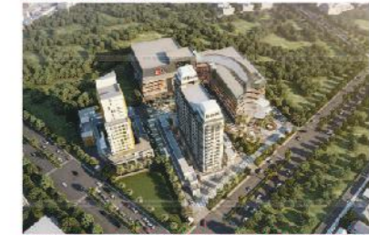
SECTOR 37 C, GURGAON-DWARKA EXPRESSWAY
