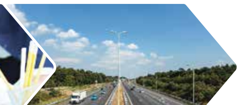
Connected with 5 Expressways
