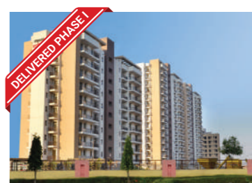
SECTOR 37C, GURGAON DWARKA EXPRESSWAY
